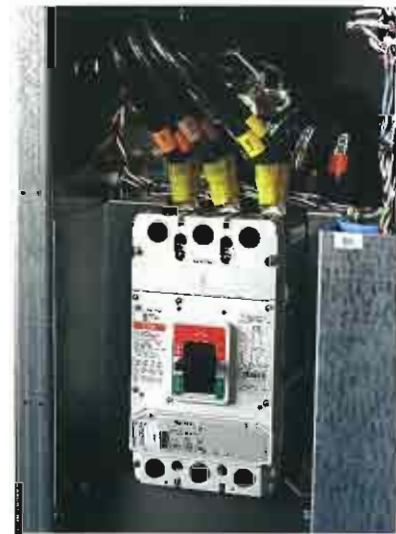
The Powerware 9395 features Cutler-Hammer LG-series input circuit breakers rated at 65 and 100 kAIC
